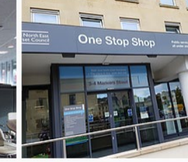
Bath and NE Somerset Council Customer Access Programme
